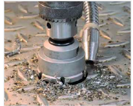
Drilling in checker sheet
